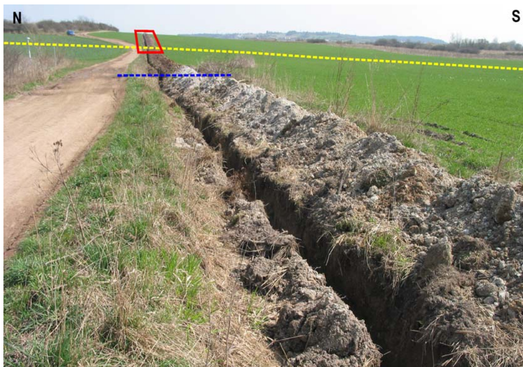
Fig. 4.8-2. Shallow trench across the basin margin south of Červený vrch hill. View at the segment 5 fault scarp from the west. Dashed yellow line shows the approximate trace of the fault zone; dashed blue line corresponds to the lithological contact Cretaceous vs. Permian-Carboniferous. Tectonic clays and cataclasites were found in the area marked by red polygon.
